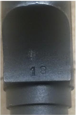
Top left photo: Although the top portion of the barrel is unmarked, 18 is stamped underneath, on the barrel flat just forward of the receiver.
